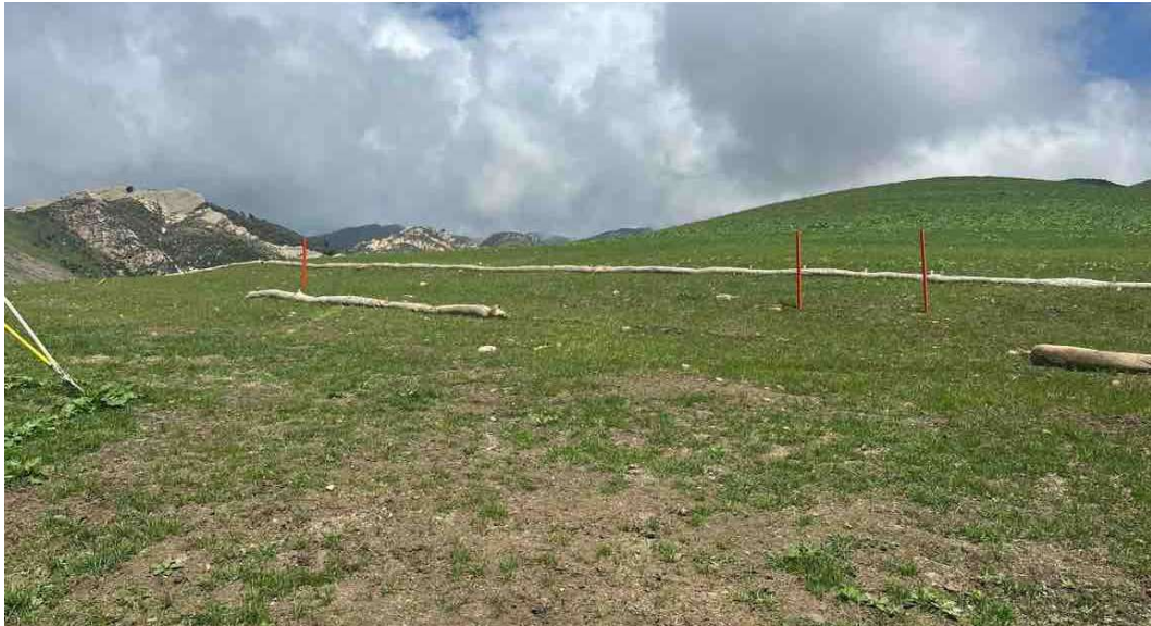
Photo 11 – Final Grading with revegetation and erosion control in place
