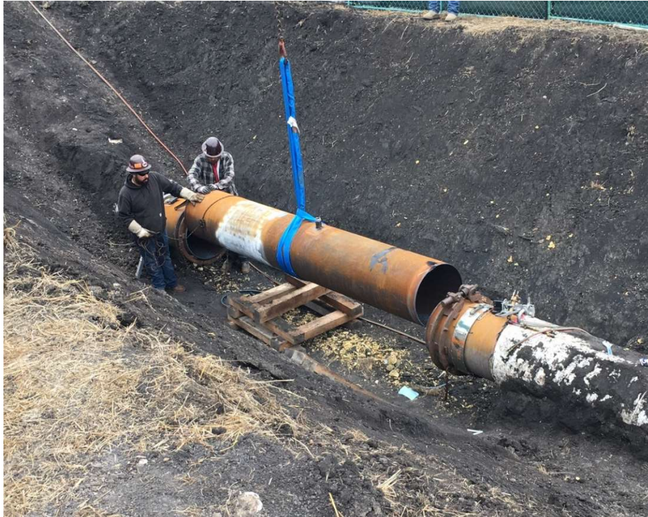
Figure 7 – Pipe Removal
