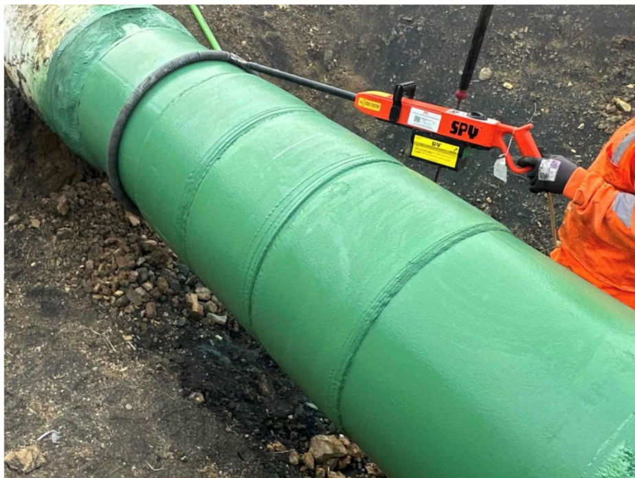
Photo 7 – Coating Inspection using a Holiday Detector “jeep”
