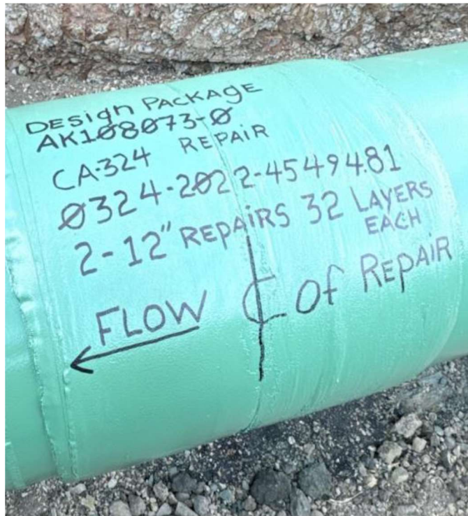
Photo 6 – Pipeline Repair – Composite A+ Wrap Cured and Initial Coating
