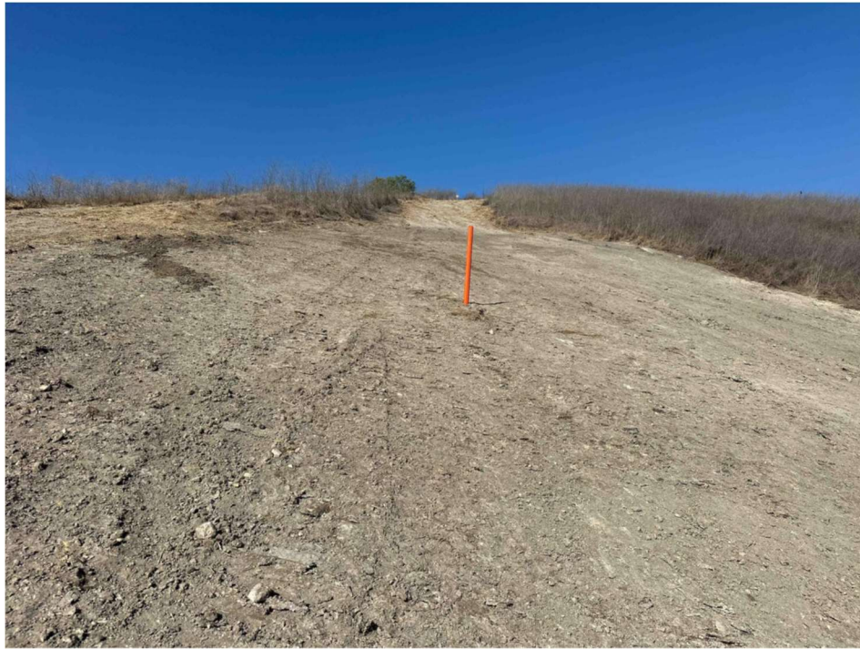
Photo 10 – Final Grading prior to revegetation with Pipeline Marker per 49 CFR 192.707
