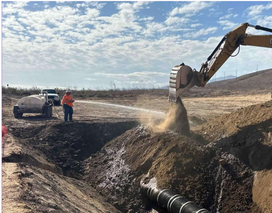
Photo 8 – A+ Wrap with final wrap post-final coating inspection prior to backfill
