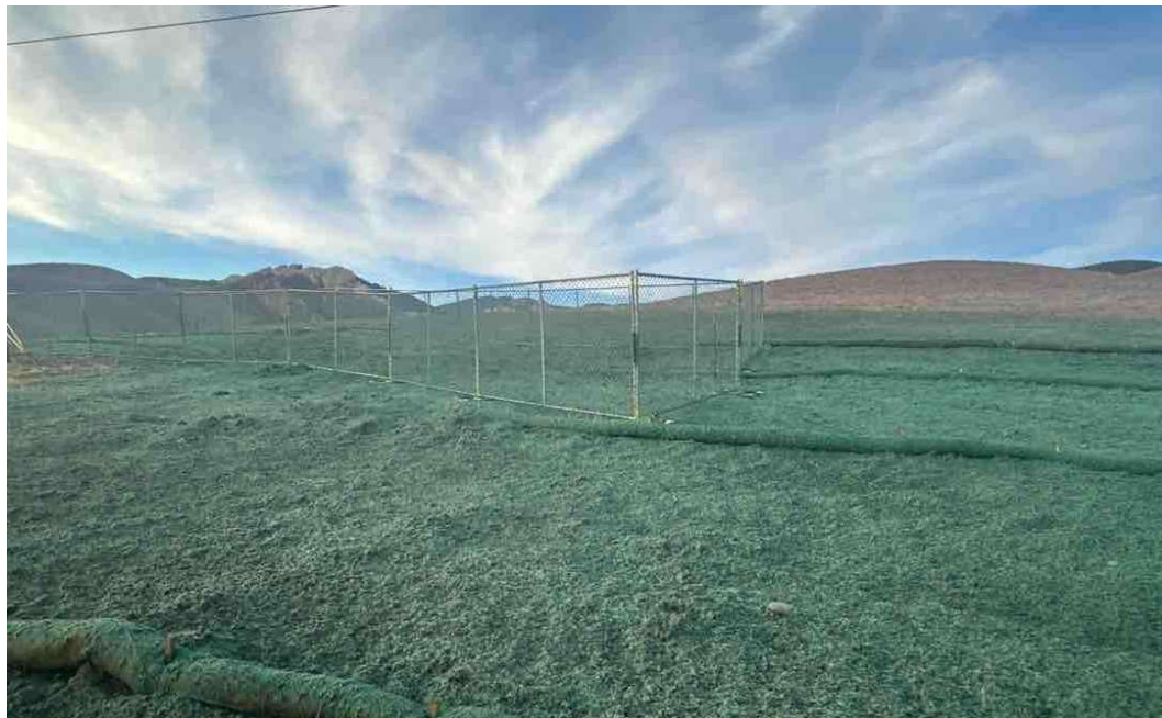
Photo 10 – Final Grading prior to revegetation with Pipeline Marker per 49 CFR 192.707
