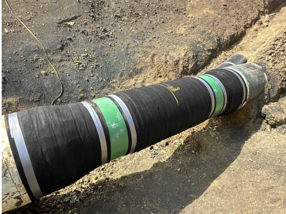
Photo 8 – A+ Wrap with final wrap post-final coating inspection prior to backfill
