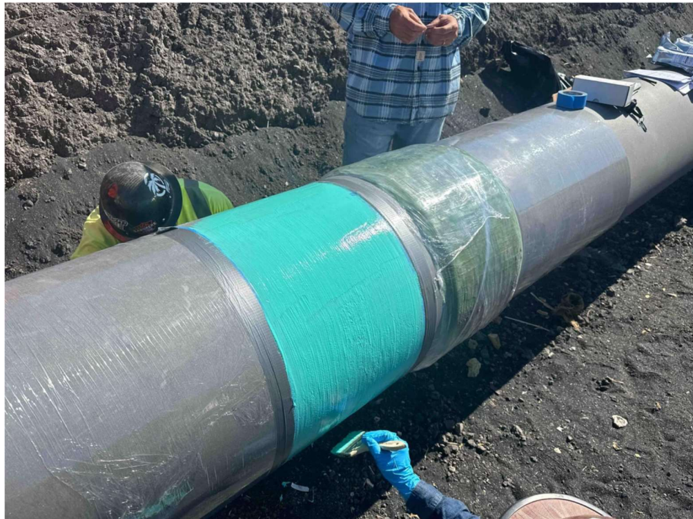
Photo 5 – Pipeline Repair – Composite A+ Wrap
