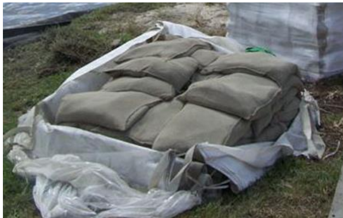
Figure 2. 3:1 Sand-to-Cement Burlap Bags
